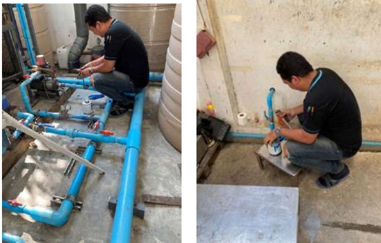
Survey to find leak water points
